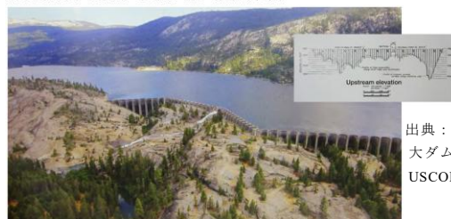
Florence Lake Dam USA California / 1926
